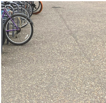
Vehicular grade asphalt with rolled buff chippings
