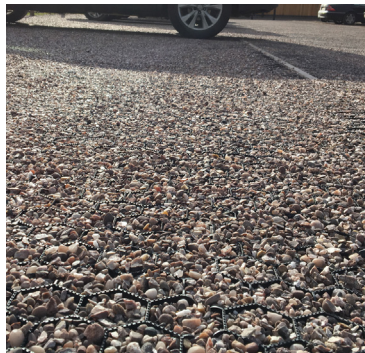
Permeable gravel retention surface
