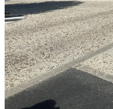
Insitu exposed aggregate concrete with sett band
